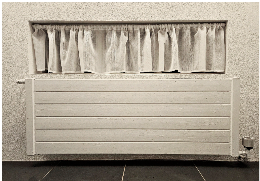
Hefðbundinn 50 ára gamall þilofn með Retúr loka, staðsettur undir glugga. – A traditional 50-year-old panel oven with a return valve, located under a window. Ljósmynd./Photo: Jónas Þór Snæbjörnsson
