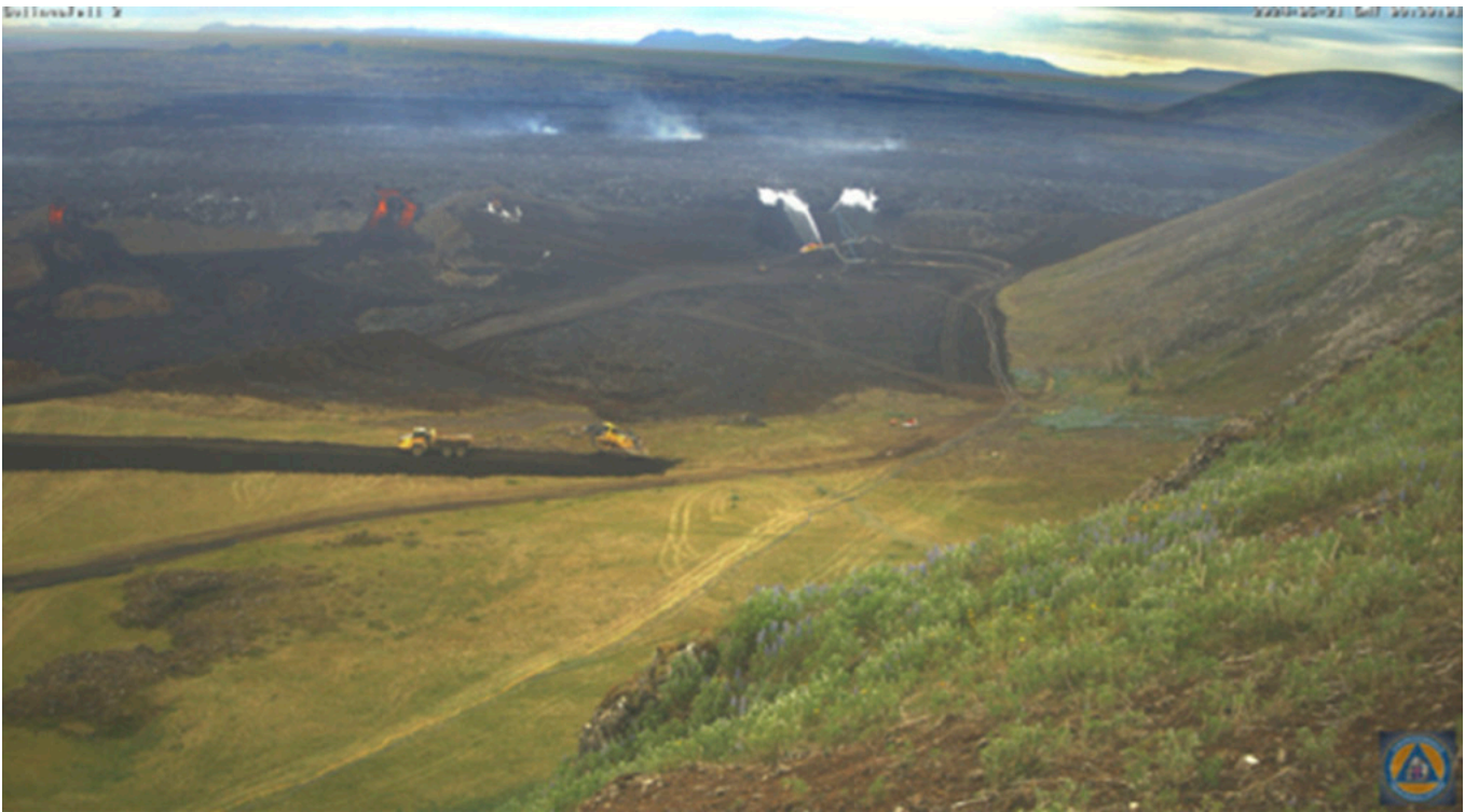
7. mynd. Vatni var sprautað á hraunjaðarinn til að hefta framgang hraunsins. – Figure 7. Water was sprayed onto the lava flow front in an attempt to slow its progression. Ljósmynd./Photo: Vefmyndavél Almannavarna – Civil Protection Authorities web-camera
