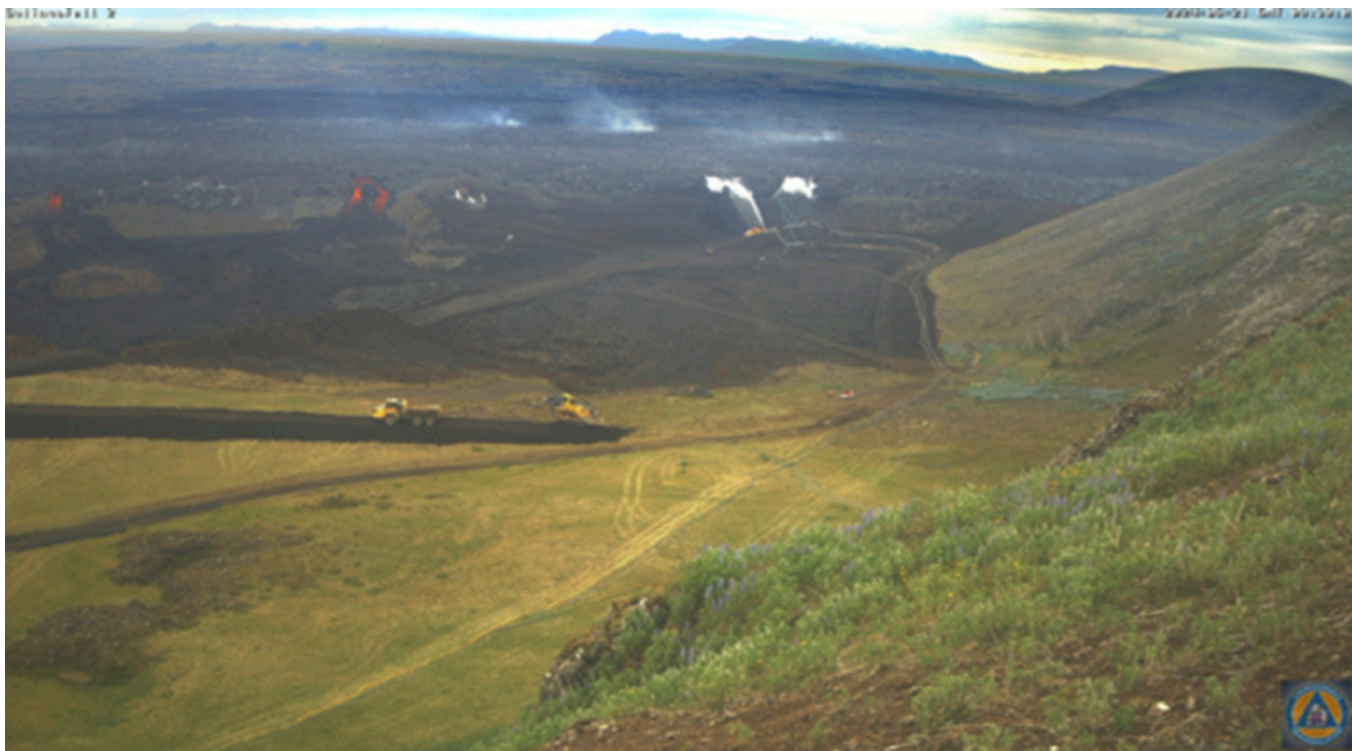
7. mynd. Vatni var sprautað á hraunjaðarinn til að hefta framgang hraunsins. – Figure 7. Water was sprayed onto the lava flow front in an attempt to slow its progression. Ljós./Photo: Vefmyndavél Almannavarna – Civil Protection Authorities web-camera
