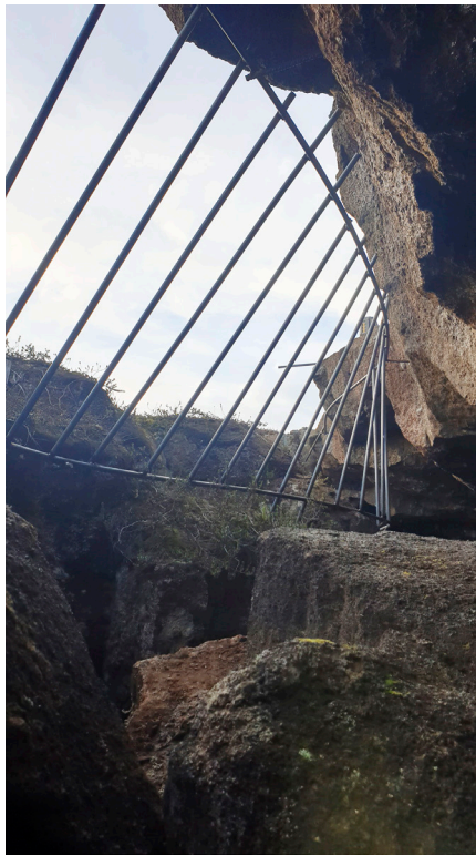
3. mynd. Stálgrind komin á hluta hellisops hellisins TES-12 í október 2020. Horft innan úr hellinum. – Half-built steel-grid cover over an entrance into TES-12 in October 2020, as seen from inside the cave. Ljós./Photo: Daníel Freyr Jónsson.
